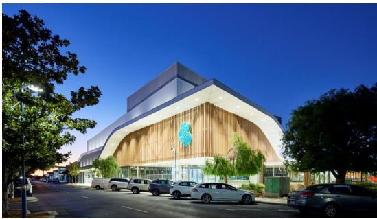
Busselton Central Shopping Centre, WA Coles, Redeveloped 2023
